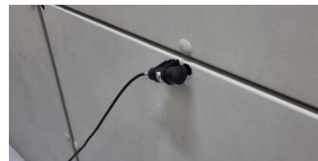
Figure 7. The external ultrasonic AA sensor is installed on the asset of interest, with the sensor head pointing through a gap between the panels.
